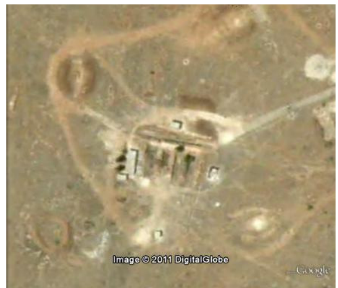
When imaged in September of 2003, the S-125 battery was no longer present at the site (Google Earth)
