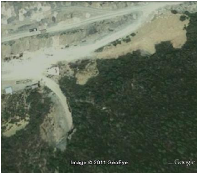
UGF complex at Bhanaka; two tunnels are under construction (Google Earth)
